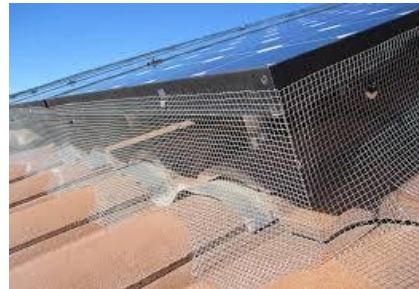
The solution – Installation of mesh screen material locked in place with clips
